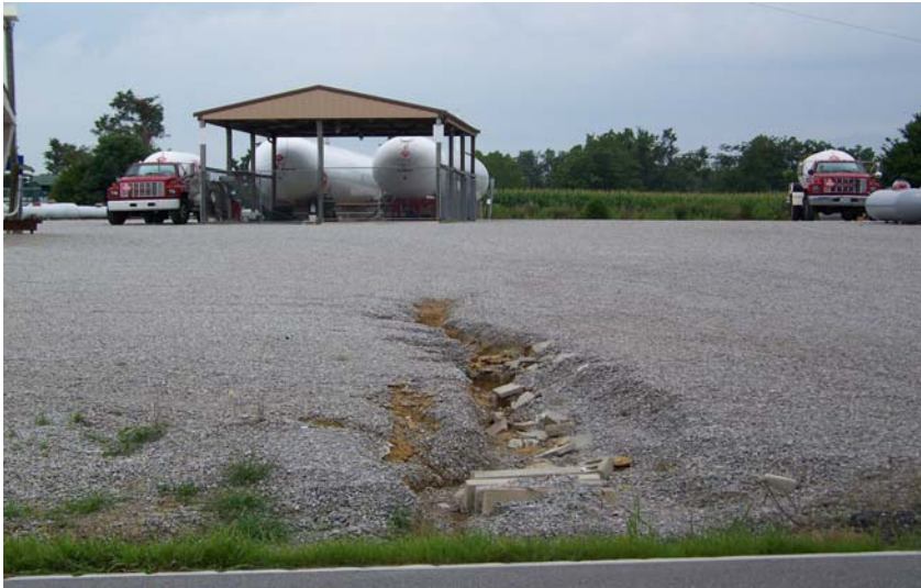
US 62 near Milepoint 24.4 in Clarkson
