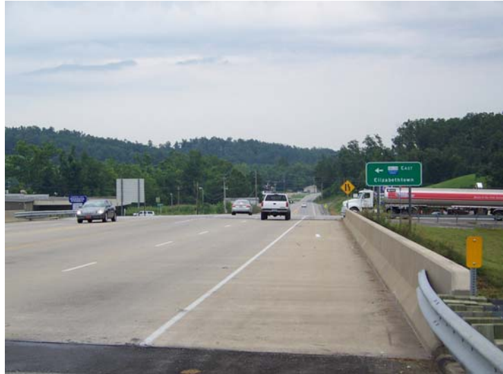
KY 259 facing South at the Western Kentucky Parkway overpass (top) and South of the Parkway overpass (bottom)
