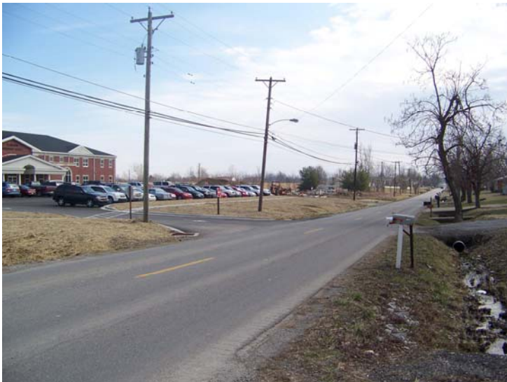
KY 224 at new Clarkson Elementary School entrance
